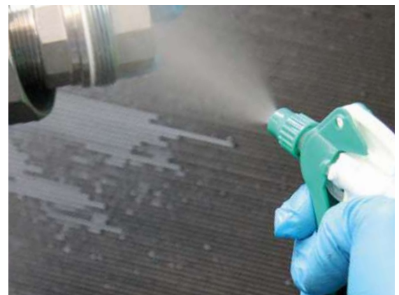
Spray on GS 200 – remove sealant
