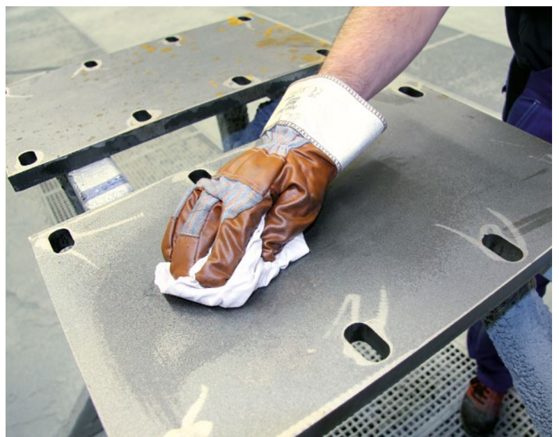
Cleaning before bonding
